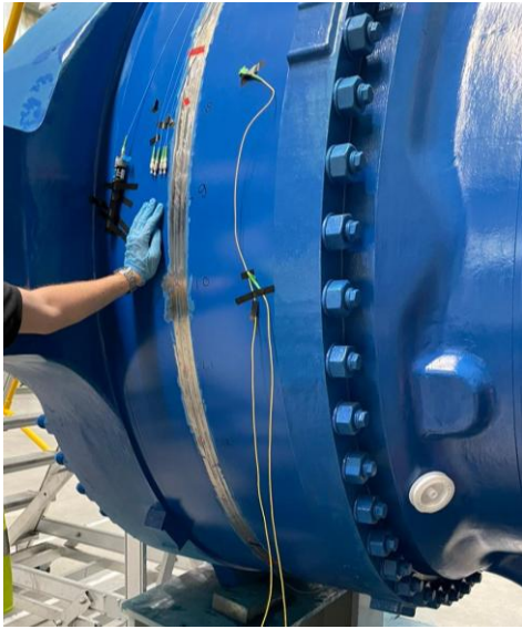
Figure 121: Installation of FBGs. Photo by Sensing 360 B.V.
